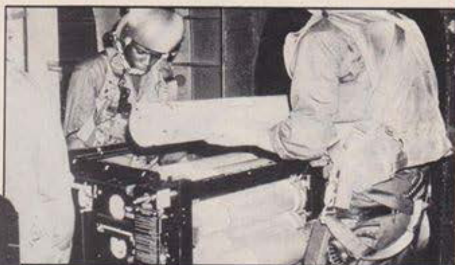
Above: Loading Mk. 24 flares into the LAU-74/A flare launcher on a Stinger. (Mike Drzyzga via Ken Wilhite)
